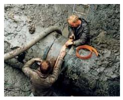
Oil & gas weld inspection using film
