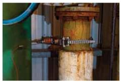
Rightrax™ permanently-installed sensor on oil & gas pipe section
